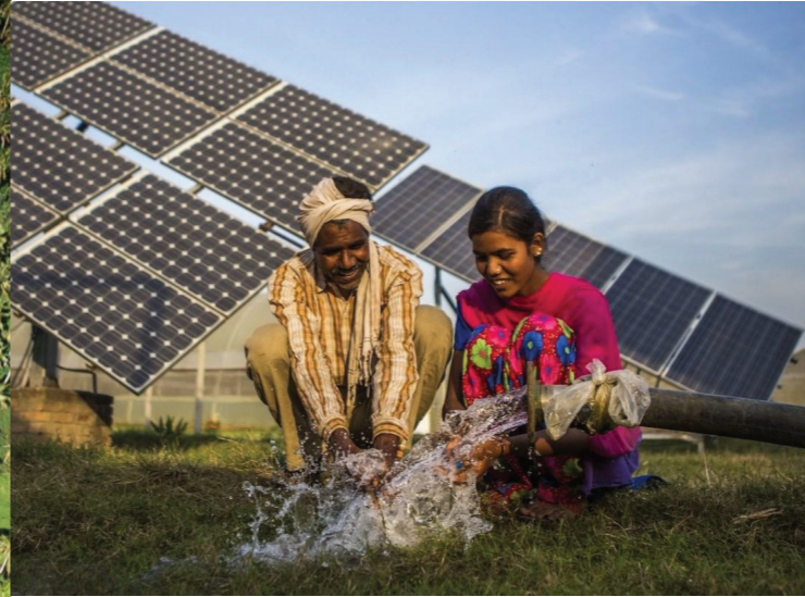
Solar Water Pumps
